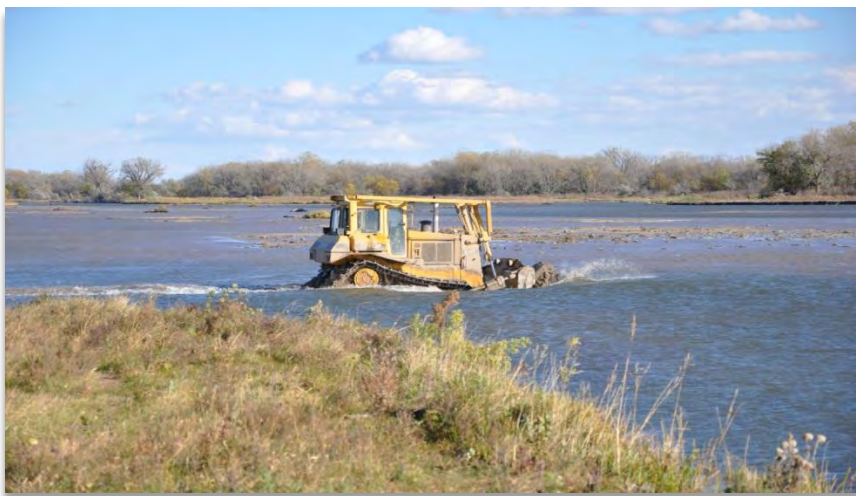
Figure 2. Typical Mechanical placement using dozers.
