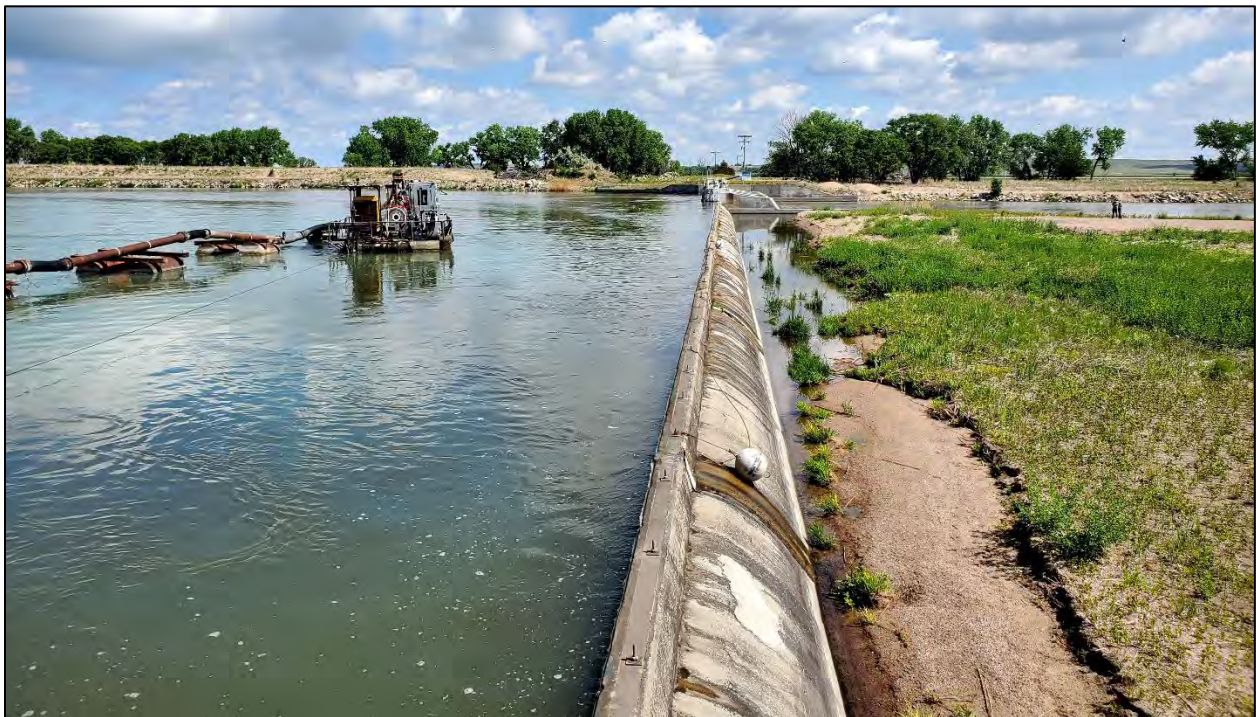
Figure 2-1. View along the crest of the Tri-County Canal Diversion Dam with active dredging operations.
